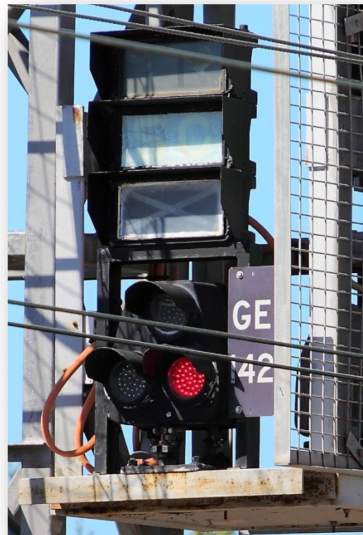
Position Light Signal with Route Indicators
