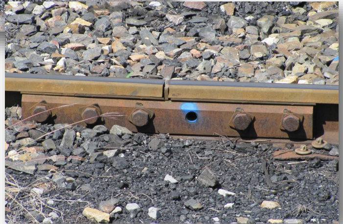
Insulated Rail Joint (Mechanical)
