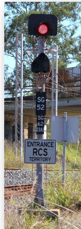
Single Aspect Red with Sub Shunt Signal
