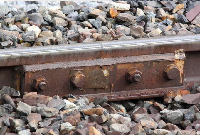
Insulated Rail Joint (Glued)
